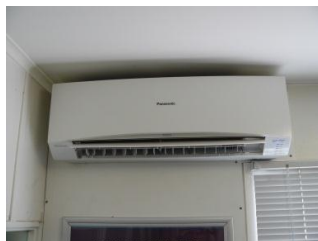
Upgrading to split system Air Conditioners
