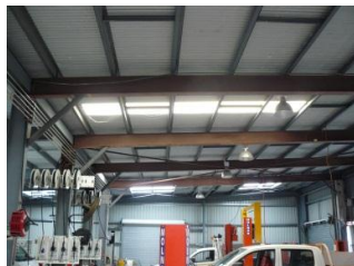
Skylights in the workshop reduce the need for lighting.
